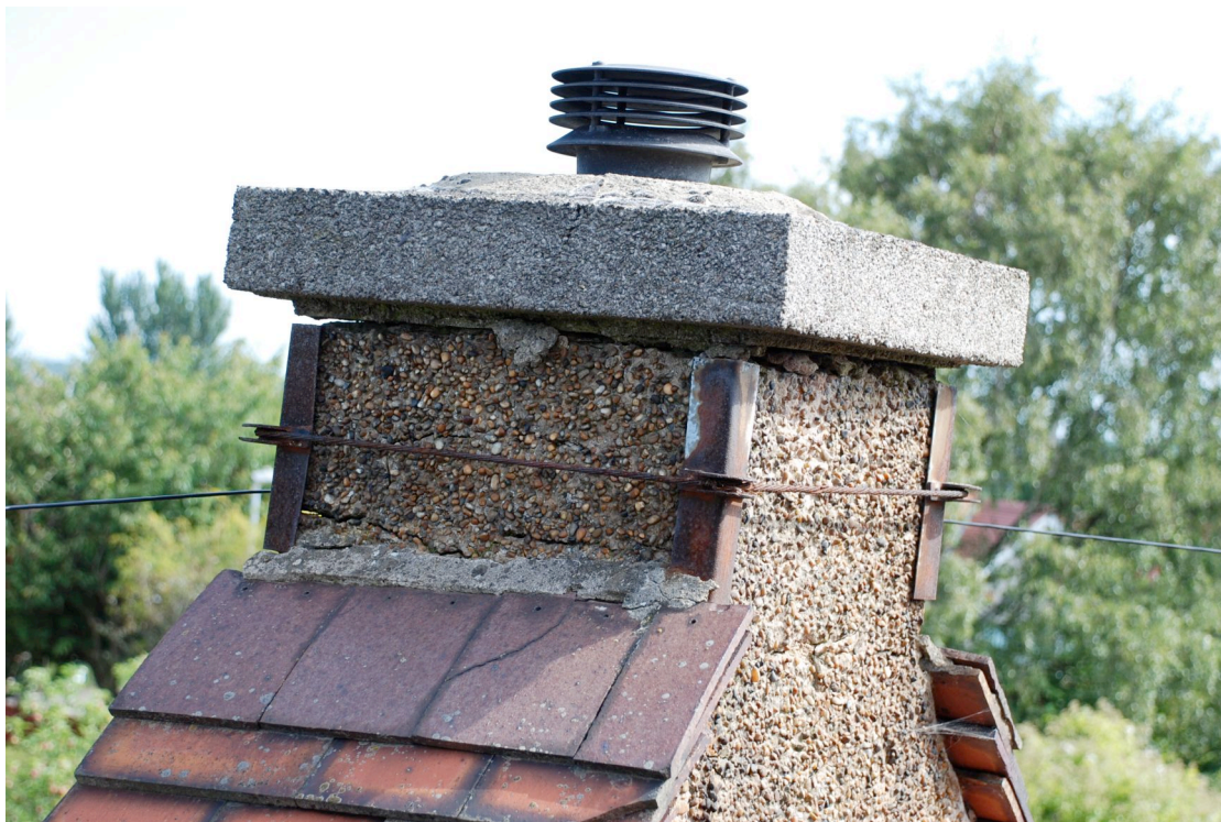
23 North east chimney, cracked render & defective pointing under cope
