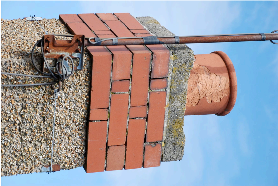
24 North west chimney, defective brick pointing & can
