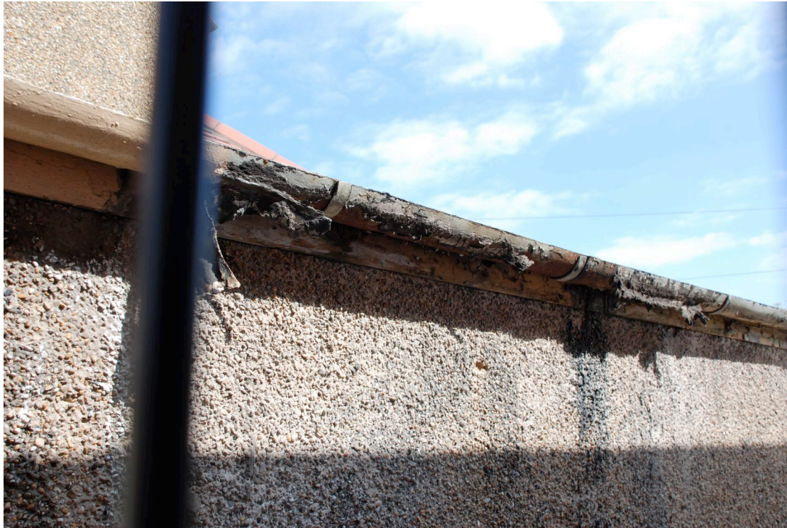
22 Defective gutter south side of garage
