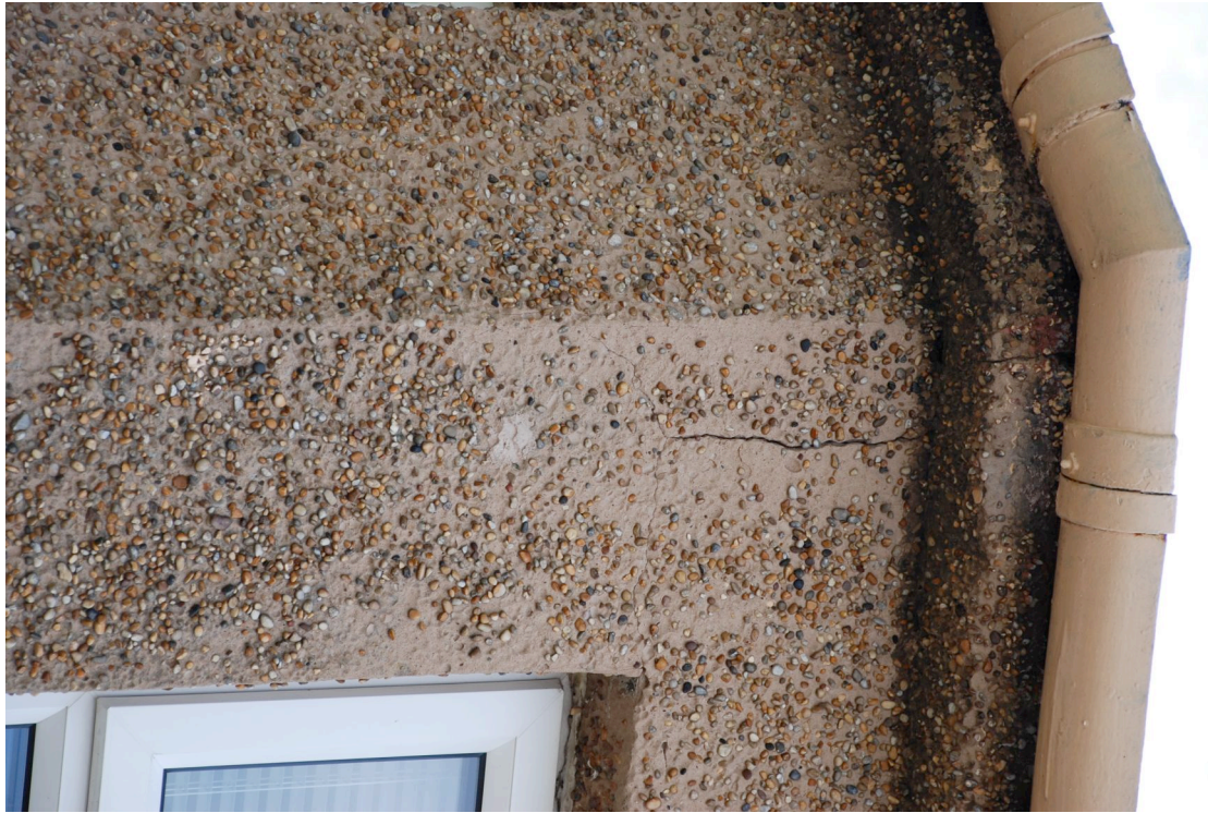
26 Front window bay, cracked render (typical)
