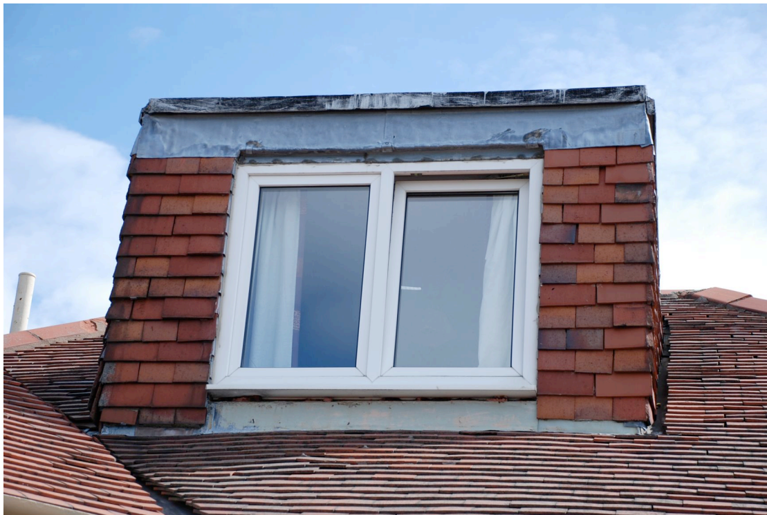
27 Front dormer, defective pointing under cill
