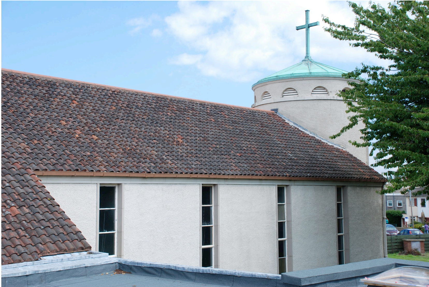
3 South Elevation of sanctuary and tower, general view
