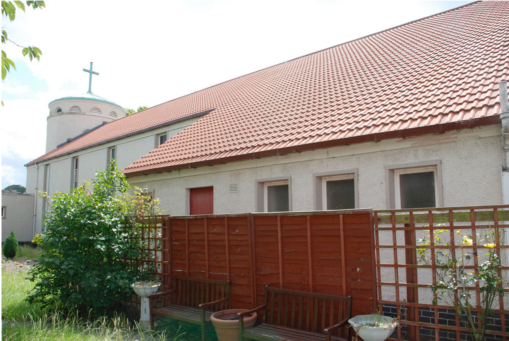
2 North Elevation, general view
