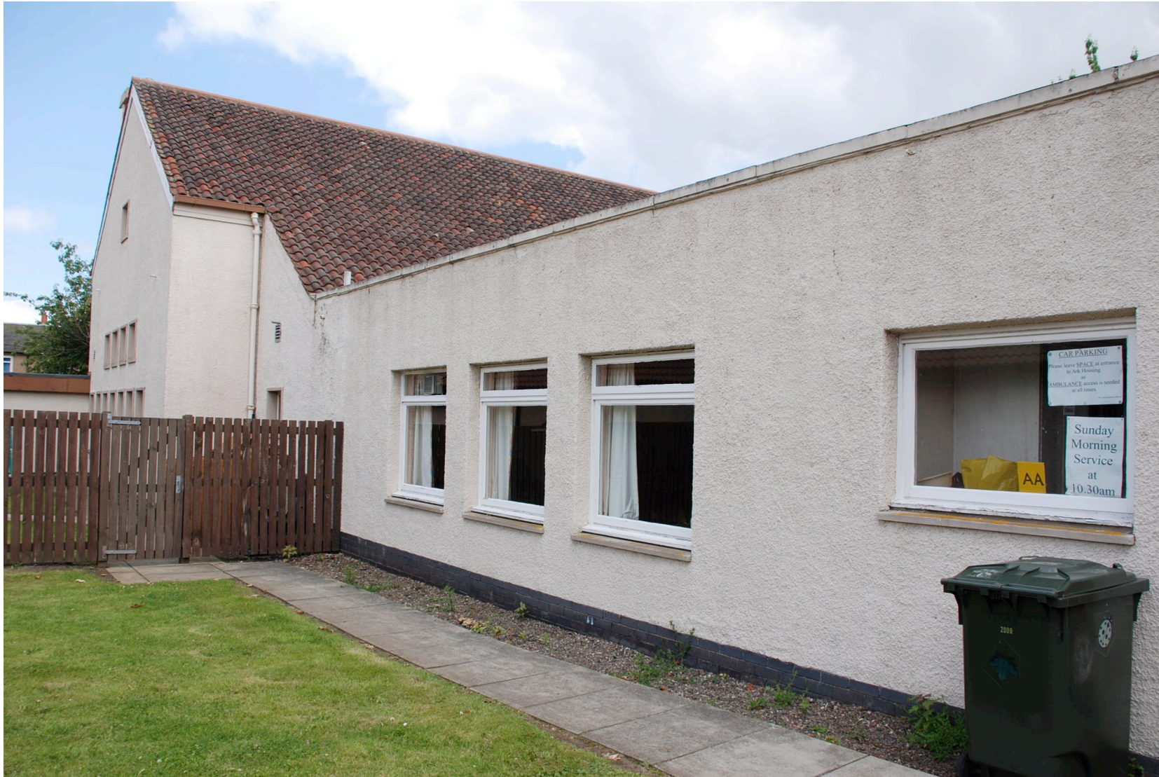
1 West Elevation, general view
