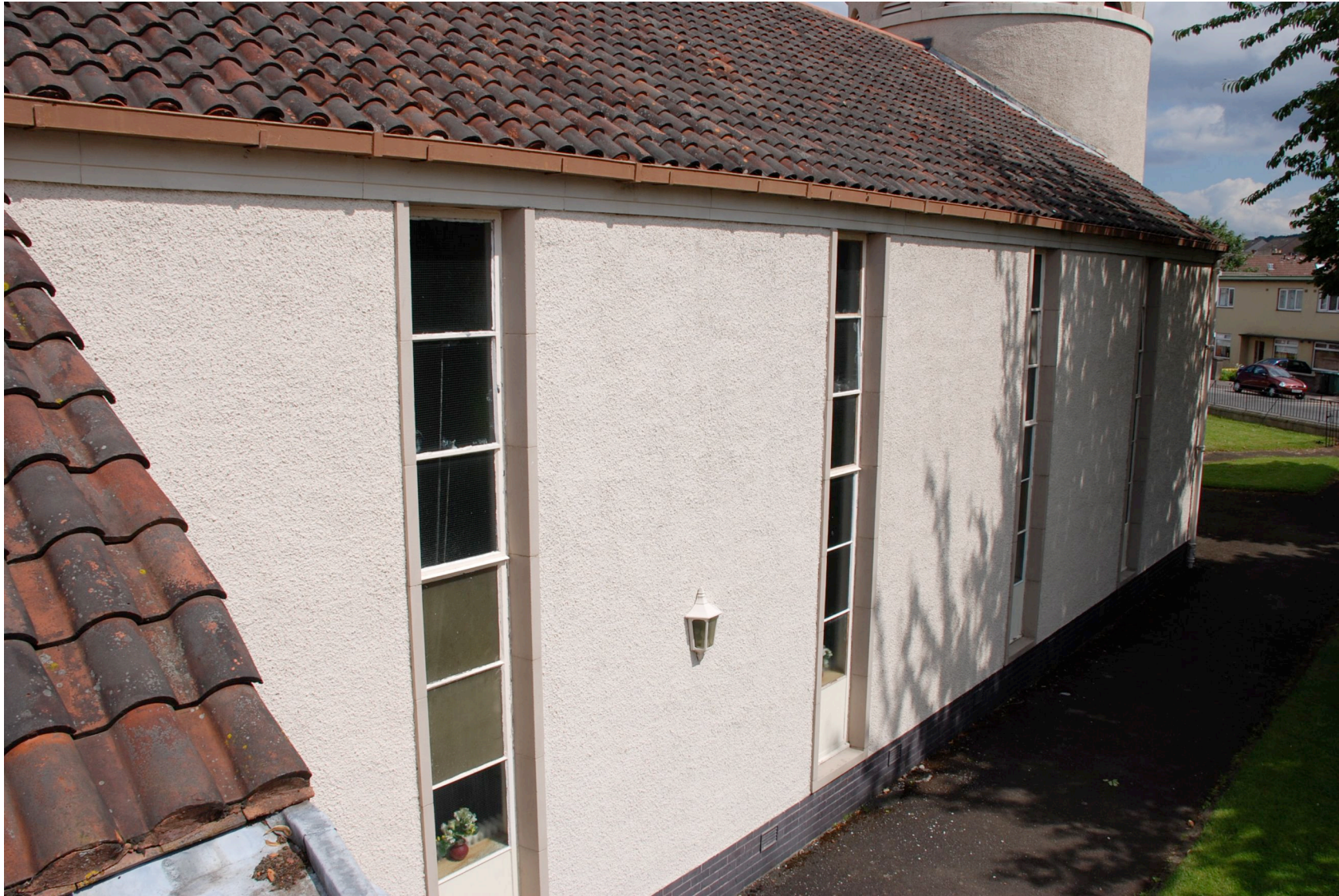
4 South Elevation, general view
